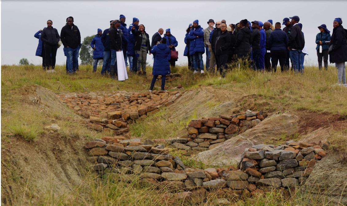
Stone bunds put in place at Ha-Lenonyane.
