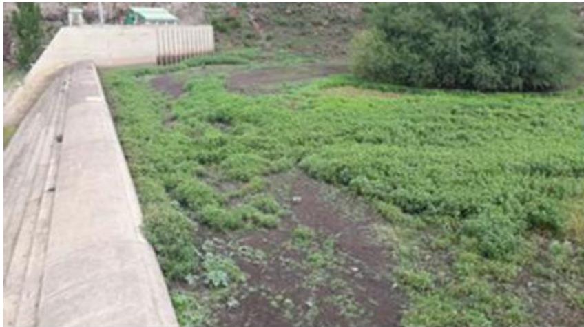
Figure 27: Matsoku Diversion Weir Siltation – May 2020 14
